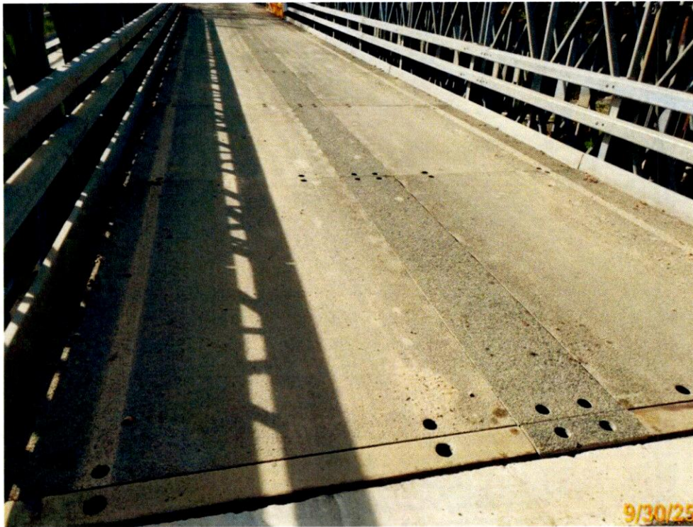
Photo 13: Wearing Surface has minor sand and debris.
