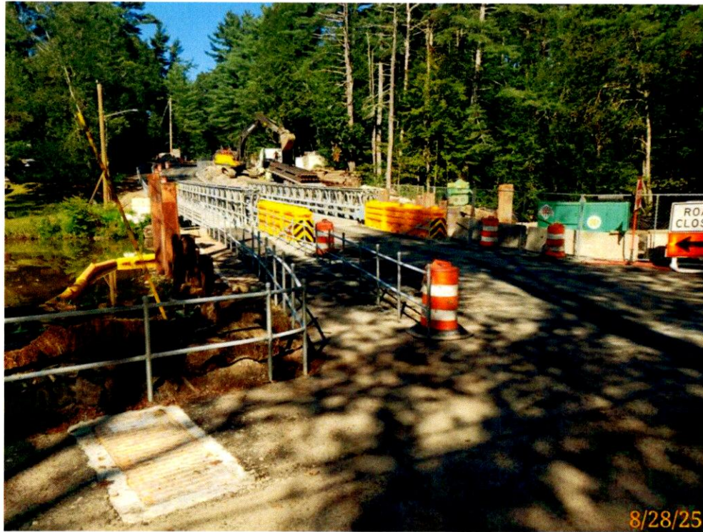
Photo 19: South Approach guardrail consists of sidewalk handrail and jersey barriers.
