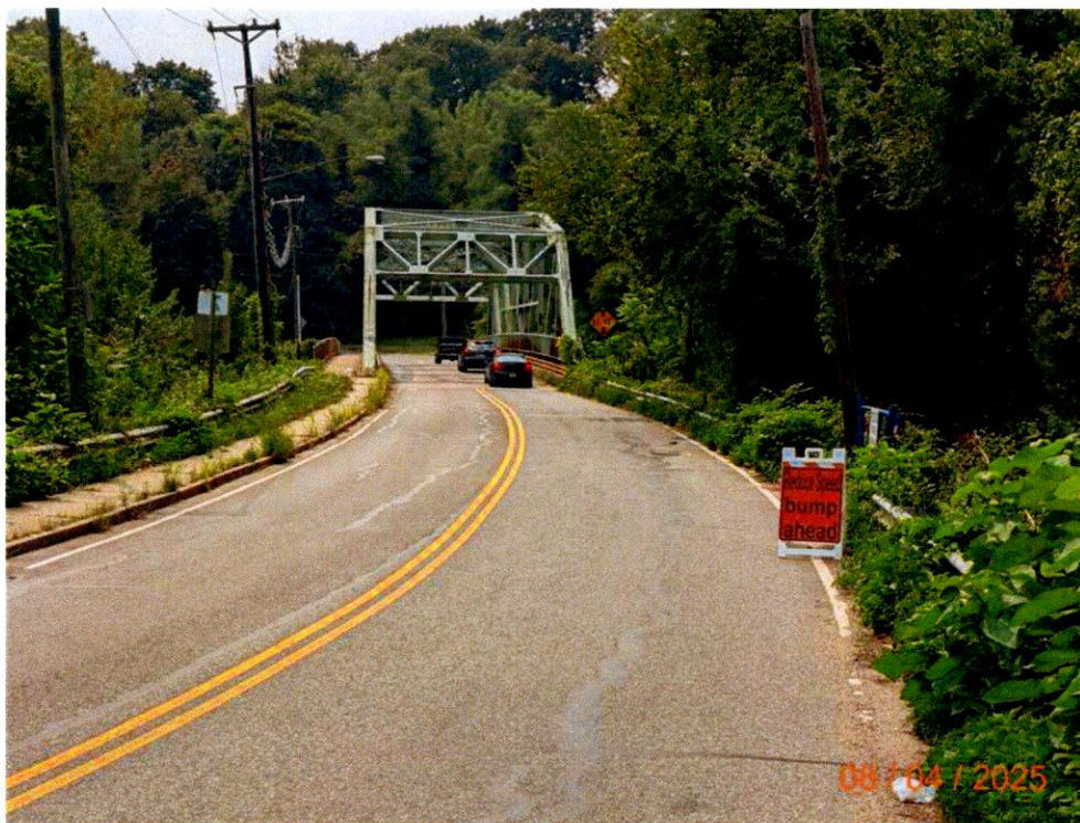
Photo 2: Signage at North Approach.
