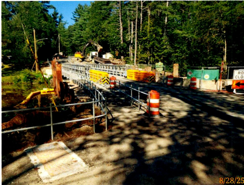
Photo 1: Pedestrian and Highway traffic is now directed onto and across the culvert. The culvert and construction site are wrapped in fencing and jersey barriers.
