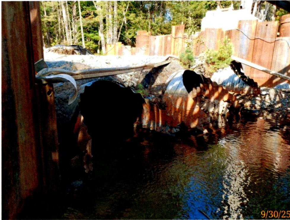
Photo 17: Scour, 0QX has been disturbed during sheet pile installation, downstream water velocity and scour has reduced significantly.
