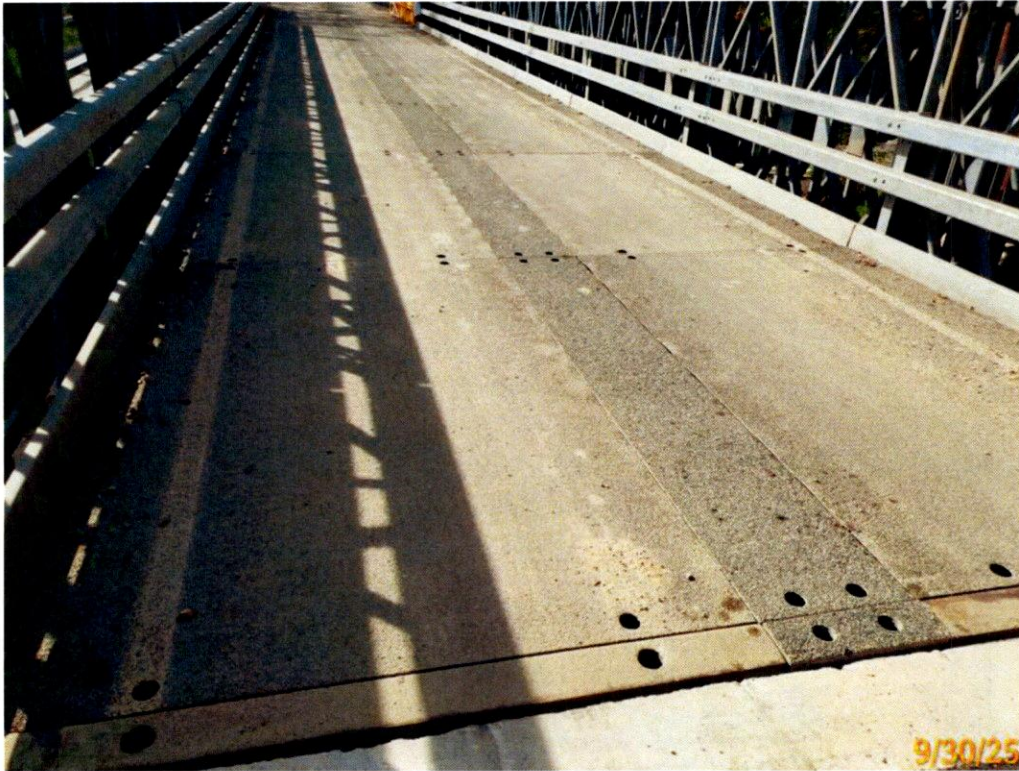
Photo 13: Wearing Surface has minor sand and debris.
