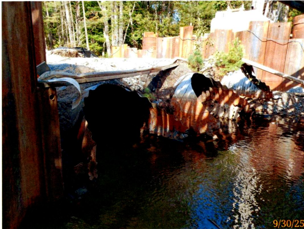
Photo 17: Scour, 0QX has been disturbed during sheet pile installation, downstream water velocity and scour has reduced significantly.
