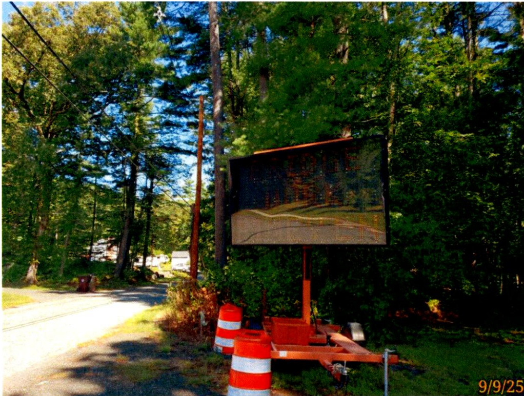
Photo 3: Advanced Signage, Alden St has 2 VMBs, the north one is not functioning.
