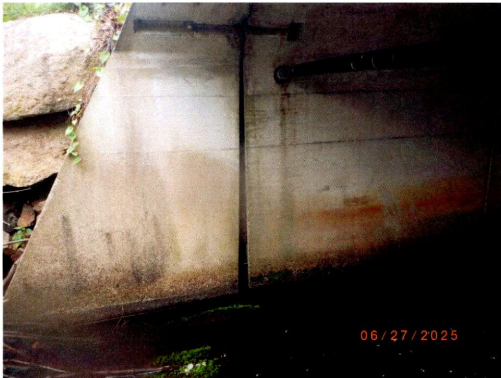
Photo 4: East Segment has separation and settlement. South side shown.
