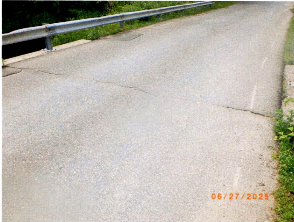
Photo 3: Wearing Surface has a transverse crack.
