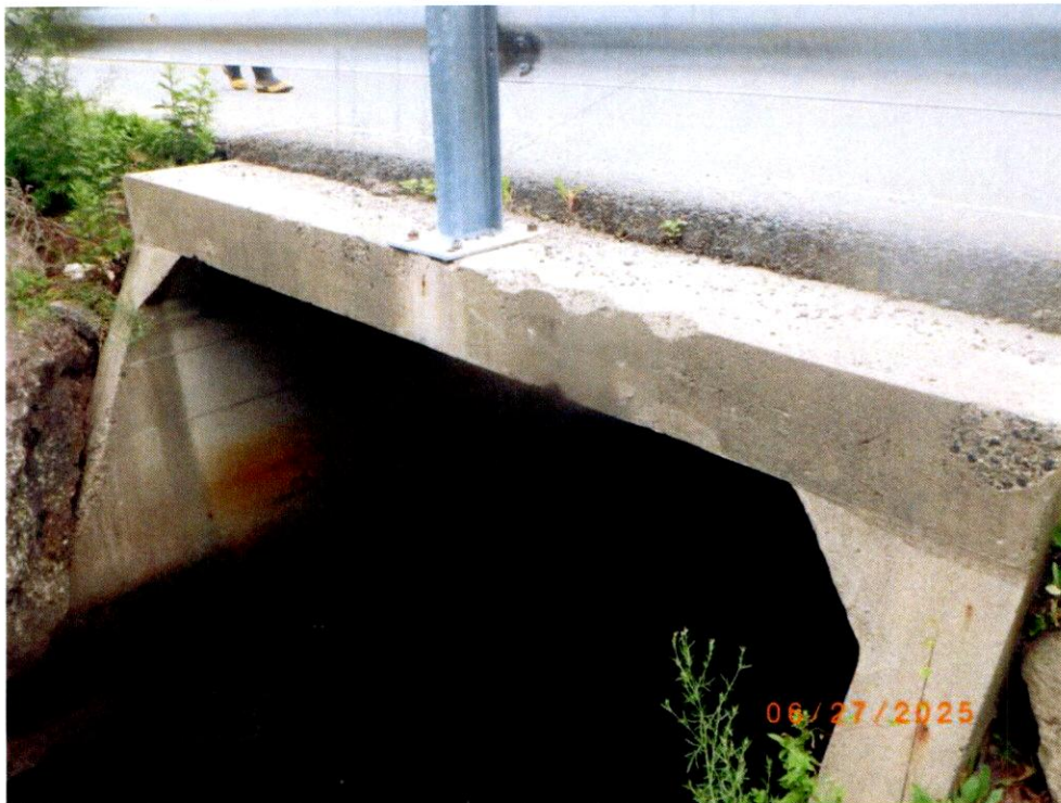
Photo 2: West Headwall has some minor chips along the top.
