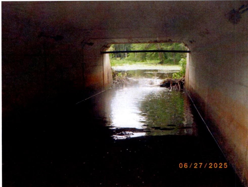
Photo 1: Roof at west segment has minor scaling with minor efflorescence, walls have waterline abrasion, segments have minor vertical misalignment, and upstream end has a beaver dam.
