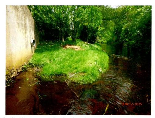
Photo 12: Upstream east elevation channel has aggradation.
