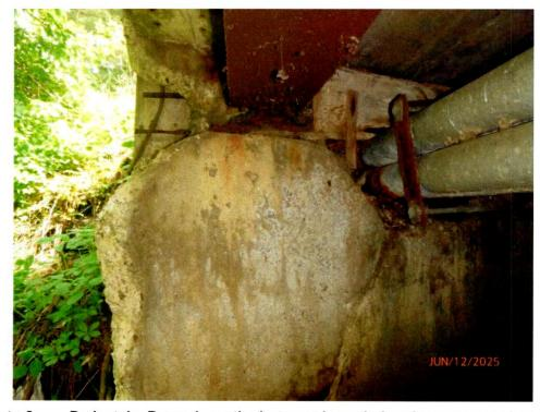
Photo 8: Pedestals, Beam 1, north abutment is scaled to the masonry plate.
