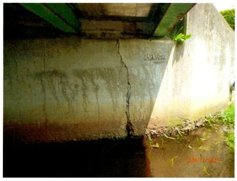
Photo 11: North Breastwall, east end has a vertical crack.
