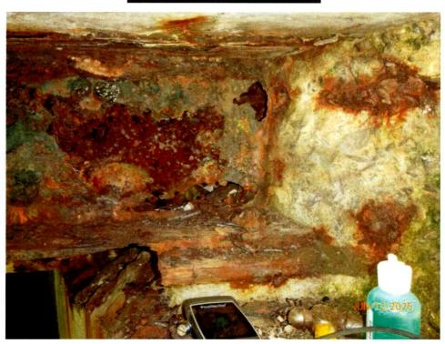
Photo 7: Beam 1, south end, east face, has holes in the web & flange.
