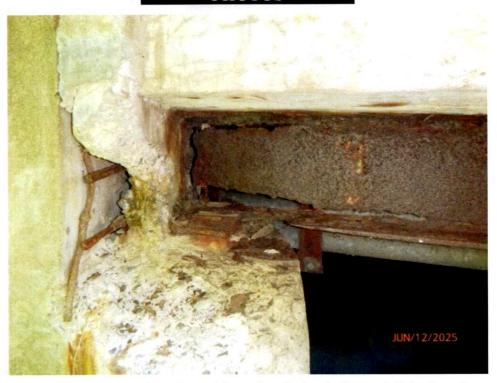
Photo 5: Beam 1, north end, west face, has holes in the web & bottom flange.
