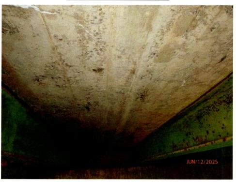
Photo 3: Interior Bays have segregation and scaling.
