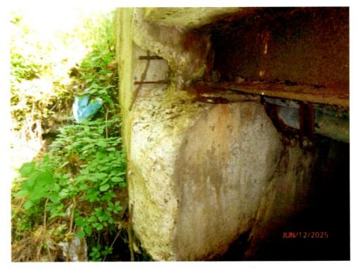
Photo 10: North Bridge Seat, west end has a large spall.
