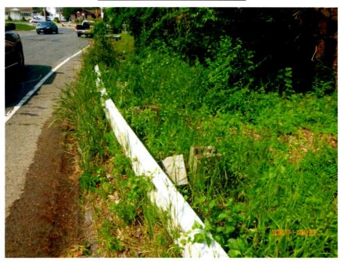
Photo 13: Northwest Approach guardrail, wood offset blocks are damaged.
