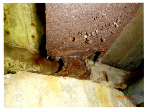
Photo 6: Beam 1, north end, bottom flange has 2 holes.
