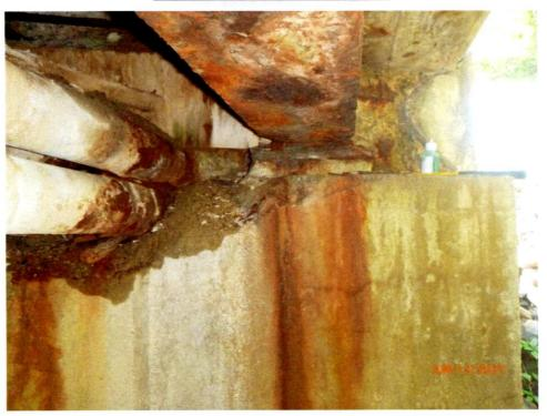
Photo 9: Pedestals, Beam 1, south abutment is scaled to the masonry plate.
