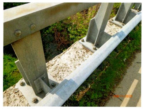
Photo 4: East Railbase has moderate scaling around the railbase plates.
