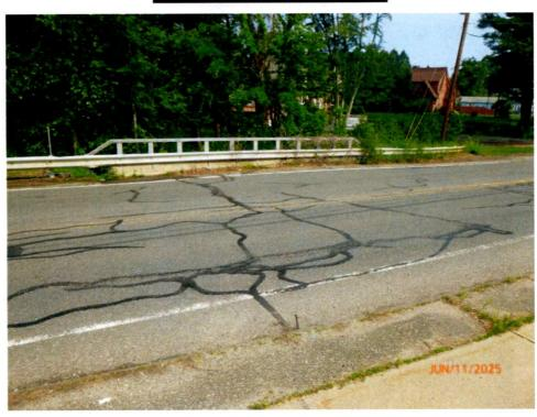
Photo 1: Wearing Surface has minor longitudinal cracking with & without crack sealant.
