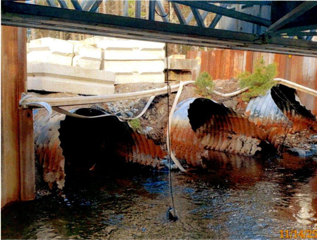
Photo 7: Scour, 0QX has been disturbed during sheet pile installation, down stream water velocity and scour has reduced significantly.
