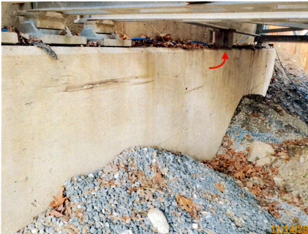
Photo 6: East Bridge Seat has minor sand accumulation. Both Bridge Seats have timber blocks that act as bolsters per the plans.
