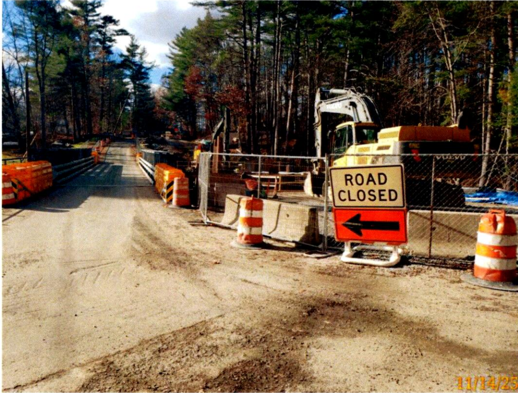
Photo 1: Pedestrian and Highway traffic is now directed onto and ACROW panel. The culvert and construction site are wrapped in fencing and jersey barriers.
