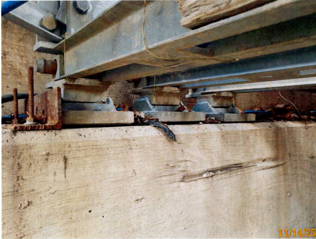
Photo 5: East Bearings (expansion) do not have anchor bolts. Each of the 3 web panels rest on an individual bearing.
