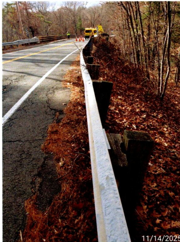
Photo 14: Northeast Approach, a few of the timber offset blocks are twisted and broken.
