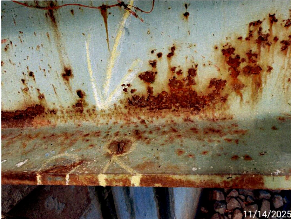
Photo 5: Beam 7, Span 1, 4.5" east of the West Bearing face, south side of bottom flange, upper face, has small laminar tears.
