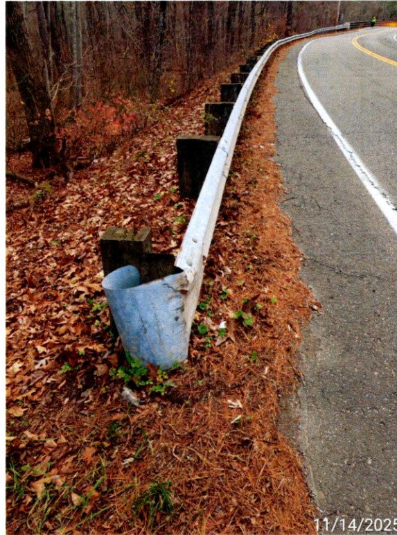
Photo 15: Southeast Approach guardrail end has minor collision damage.
