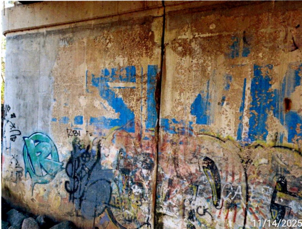
Photo 11: East Breastwall, around the center construction joint, spalled and delaminated.
