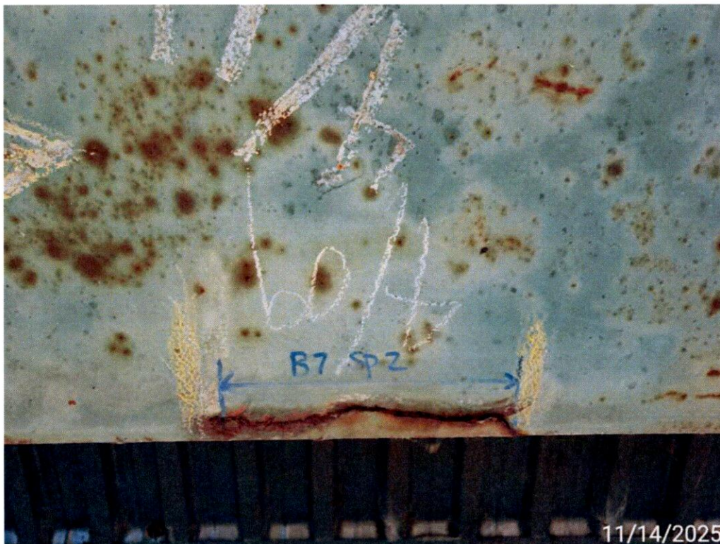
Photo 6: Beam 7, Span 2, 8' east of Diaphragm 2, north side of bottom flange, lower face has a laminar tear.
