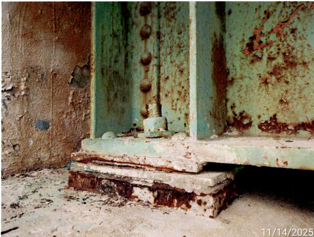
Photo 8: Some West Abutment bearings have pack rust between the sliding plates and the masonry and sole plates. A few of the anchor bolts are bent. (Bearing 7 shown.)
