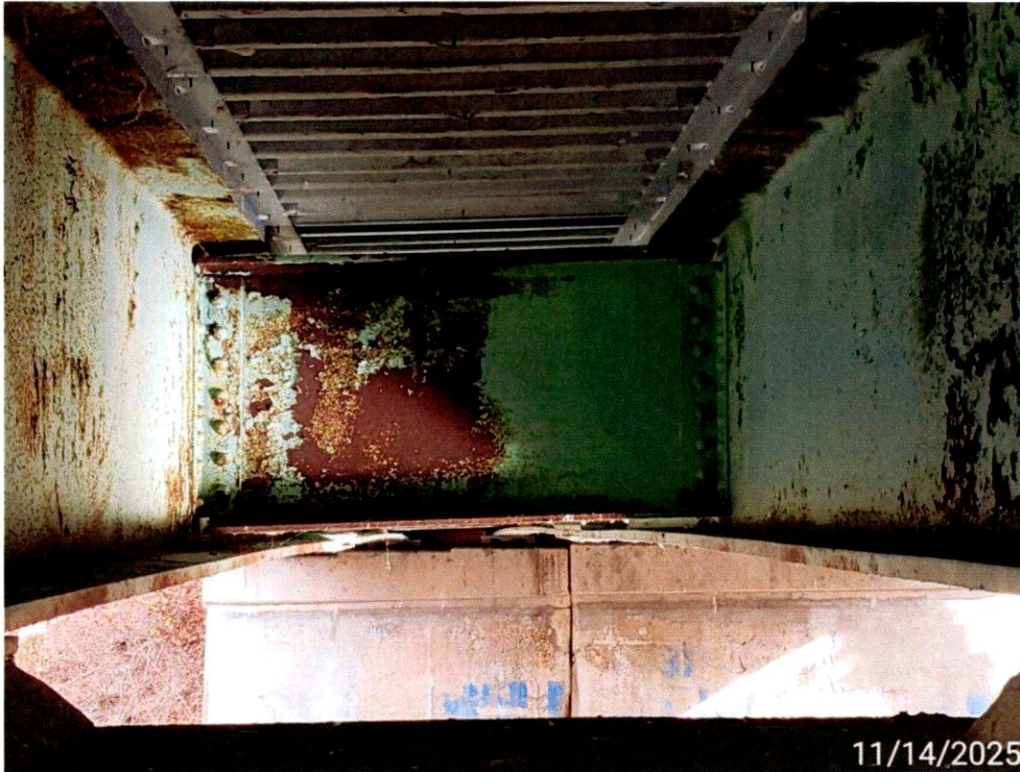
Photo 9: Some of the Steel Diaphragms have minor to moderate surface rust.
