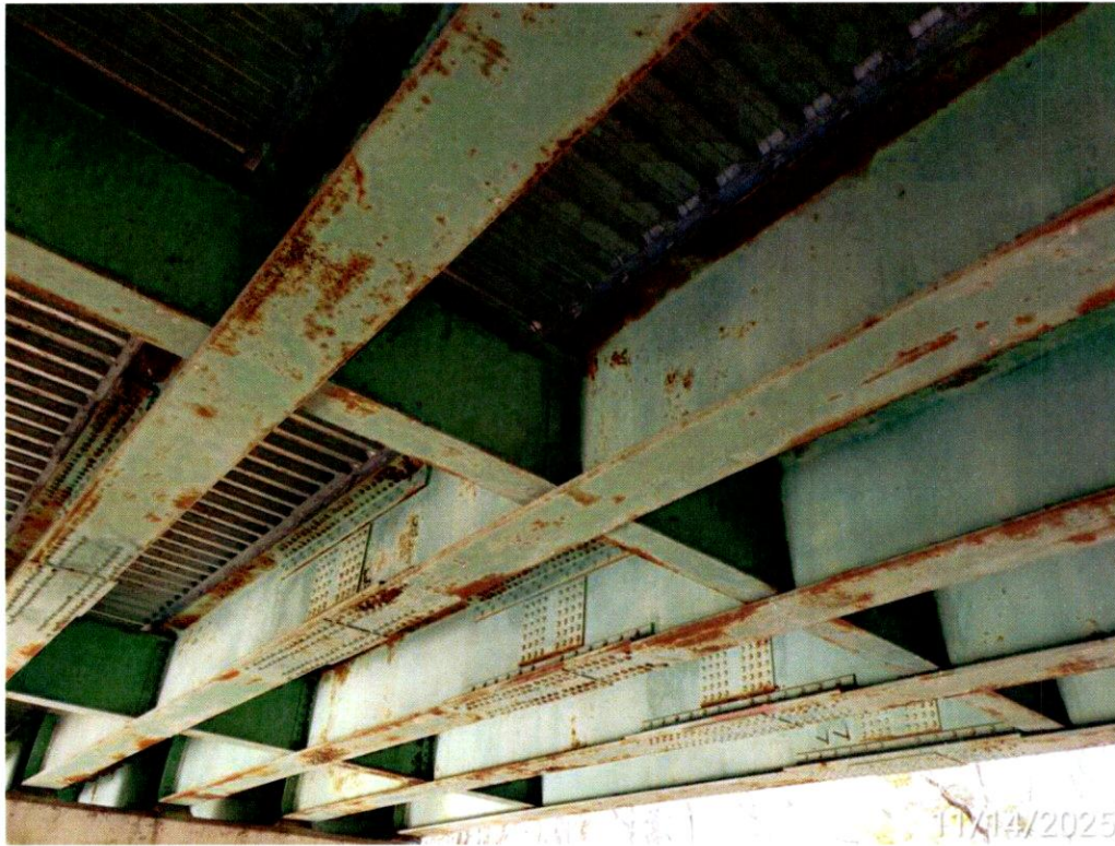
Photo 7: Riveted connection plates have minor to moderate surface rust.
