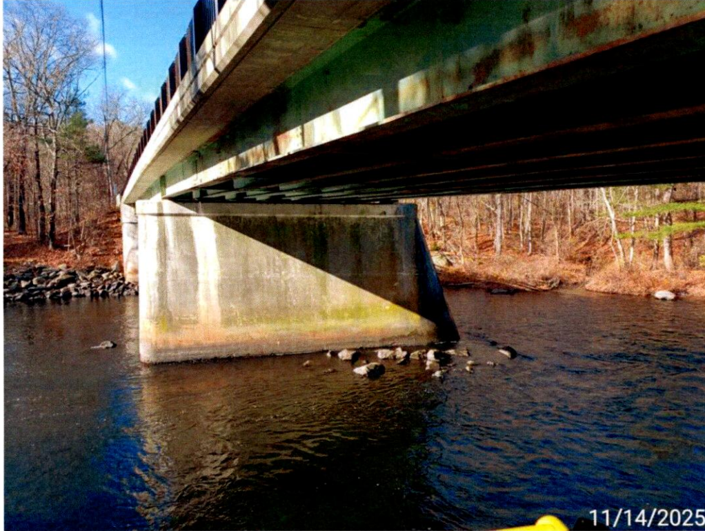
Photo 13: Downstream half of the Pier Stem Base, on both sides, has areas of scaling.
