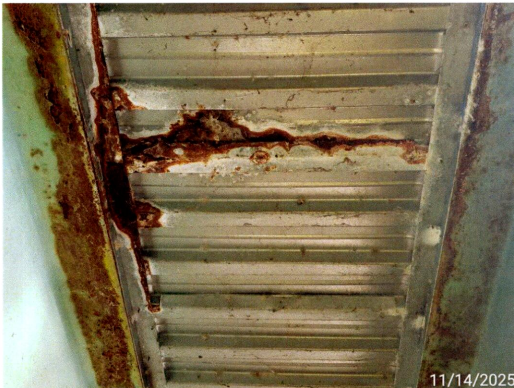
Photo 2: Stay-In-Place Form, Span 1, Bay 6, East of Diaphragm 3, one area of surface rust with one rust hole, exposing solid concrete.
