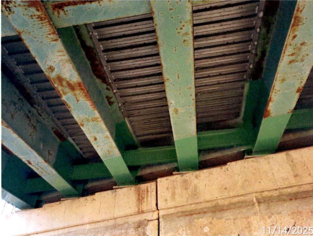
Photo 1: East Abutment has reconstructed Bridge Seat, Backwall, & Concrete End Diaphragms. East Beam Ends and steel end diaphragms are repainted.
