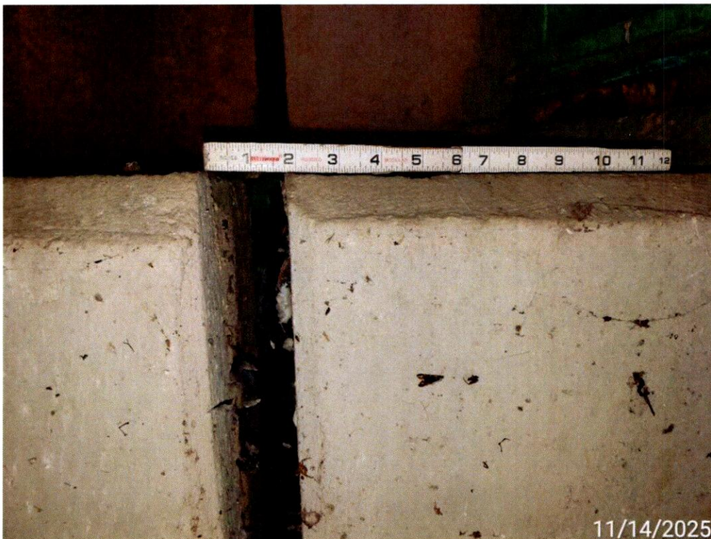
Photo 12: West Breastwall, settlement, the gap at the construction joint.
