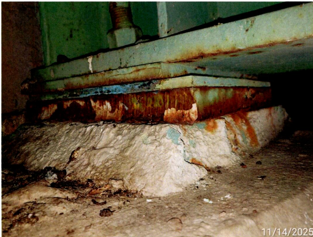
Photo 10: West Bridge Seat, concrete pedestal east face for Beam 4 is spalled.
