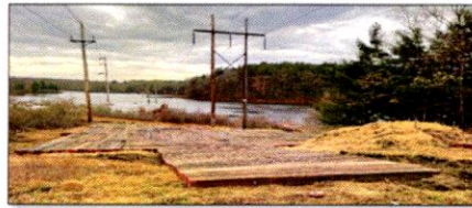
Timber mats "matting"
