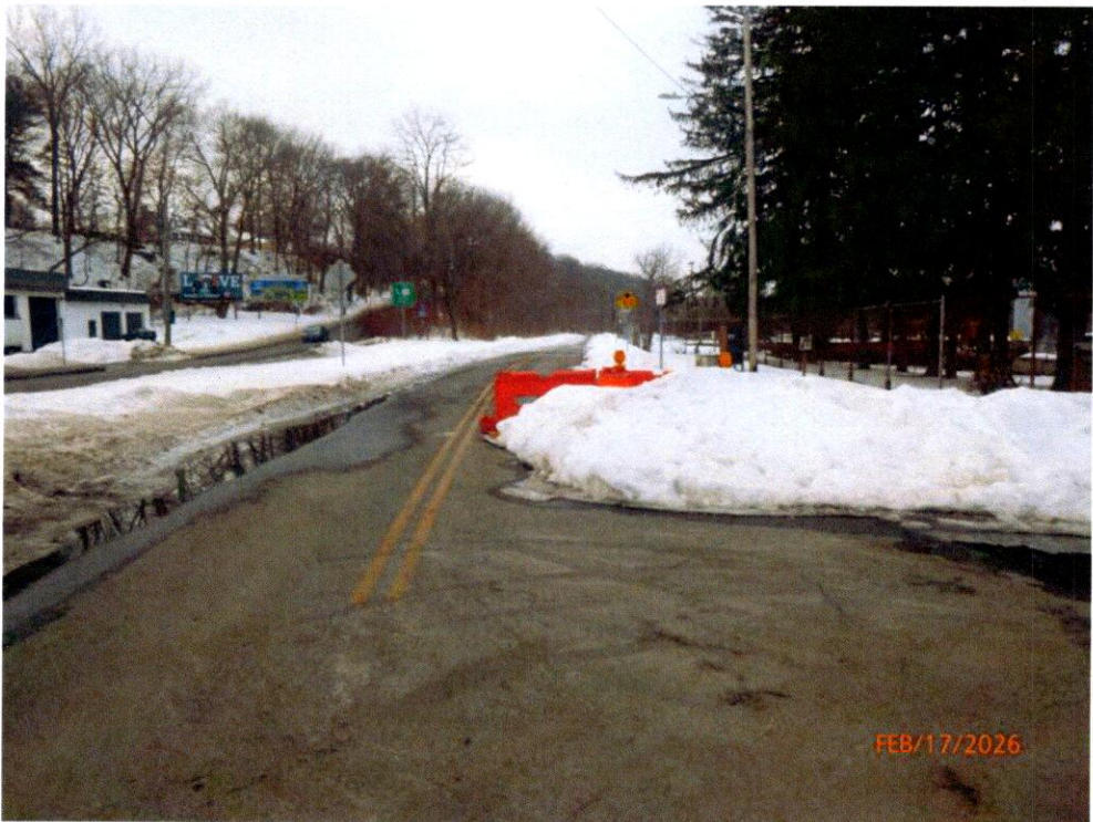
Photo 2: South Advance Warning: Road Closed Sign, Barrels, and Barriers are partially to fully buried in snow.
