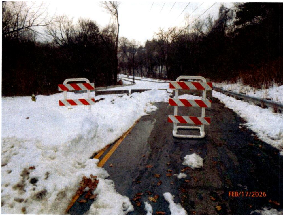
Photo 5: North Advance Warning: 2 Hazard Barriers & 3 concrete barriers partially buried in snow, 500' north of bridge.
