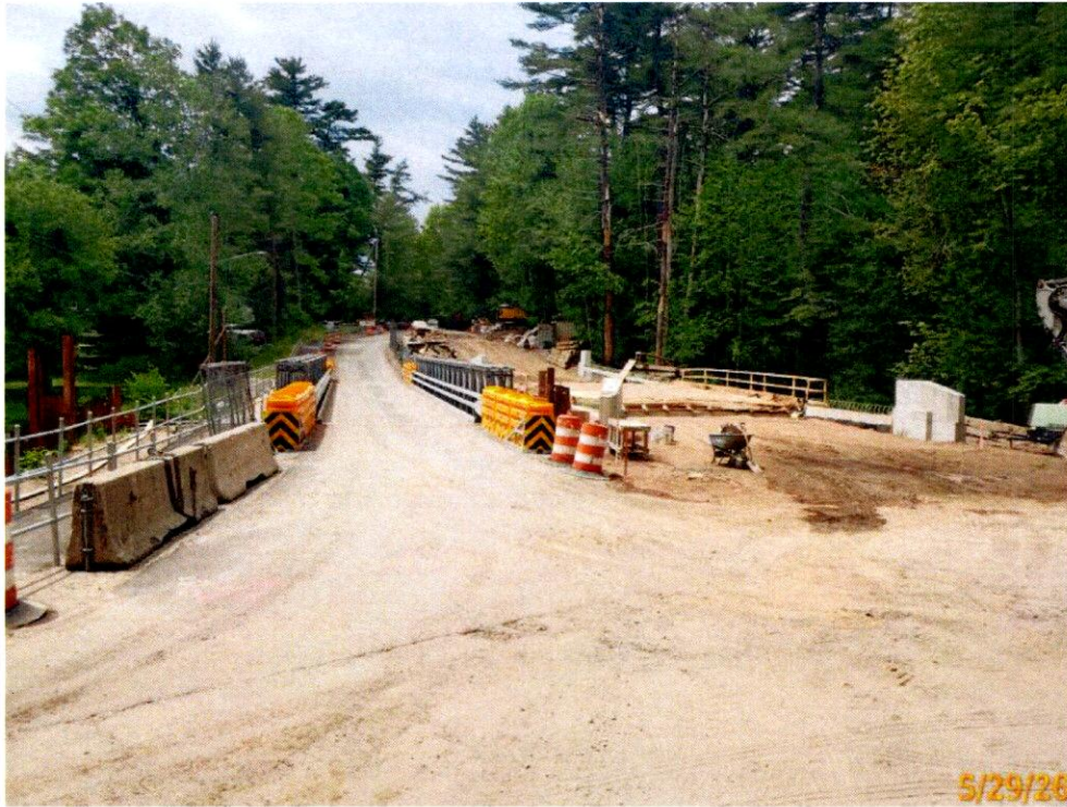
Photo 1: Pedestrian and Highway traffic is directed onto and ACROW panel. The construction site has barriers removed during active construction.
