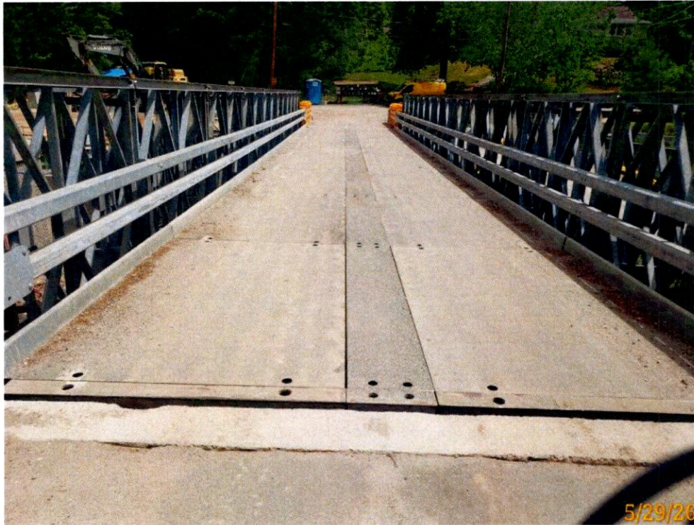
Photo 5: Wearing Surface has minor sand and debris.
