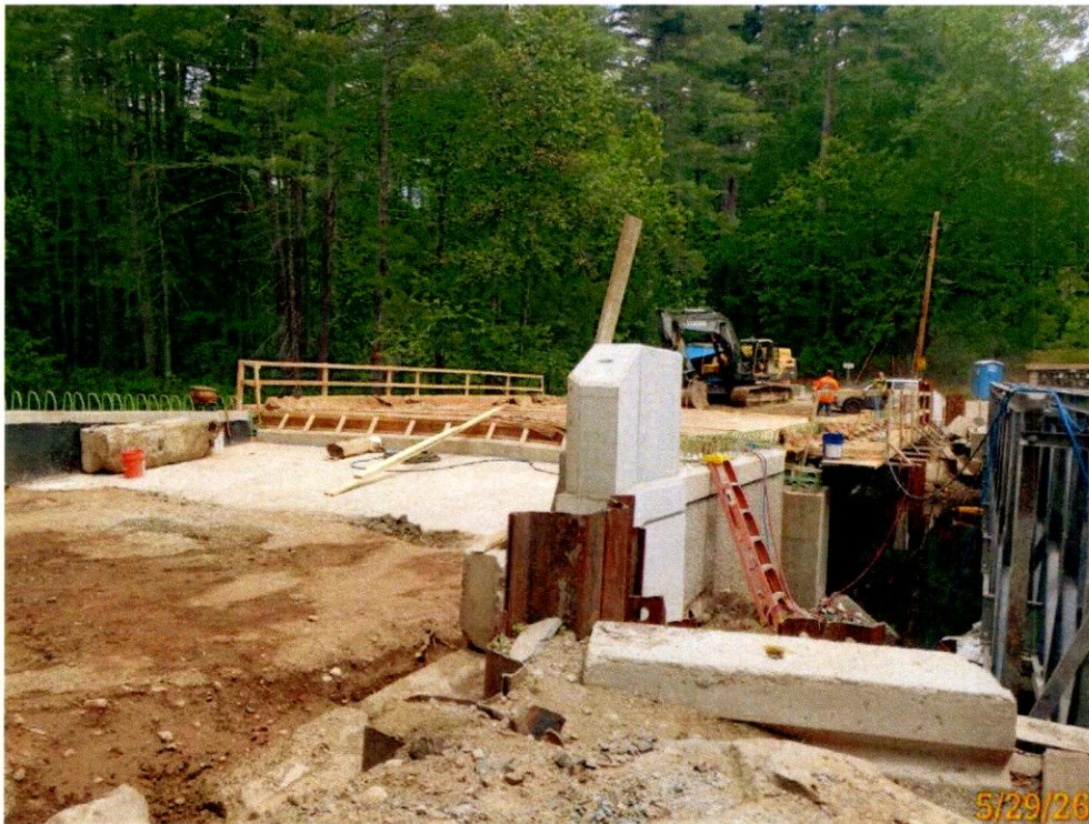
Photo 2: Since the last inspection, the culvert has been fully removed.
