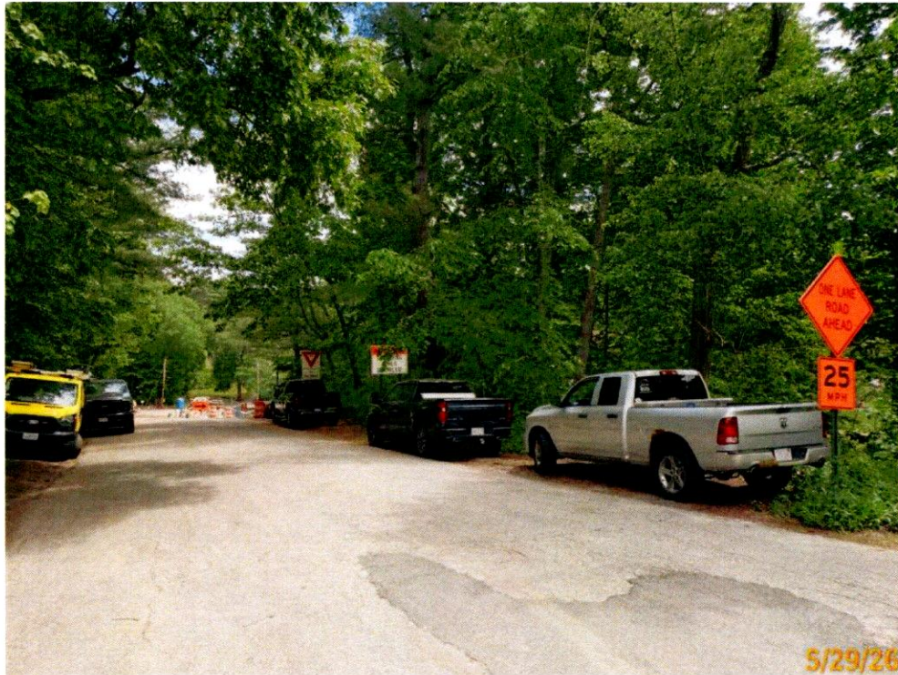
Photo 3: West Advanced Signage, typical condition.
